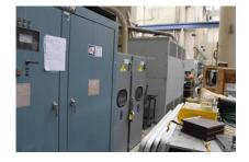
**Available Power** - In addition to various bench top instrumentation power supplies, CEM also has a 250 Volt 6,000 Amp de power supply located in the main high bay. 4160 V available in the second story transformer vault, with 480 V available throughout the high bay.
